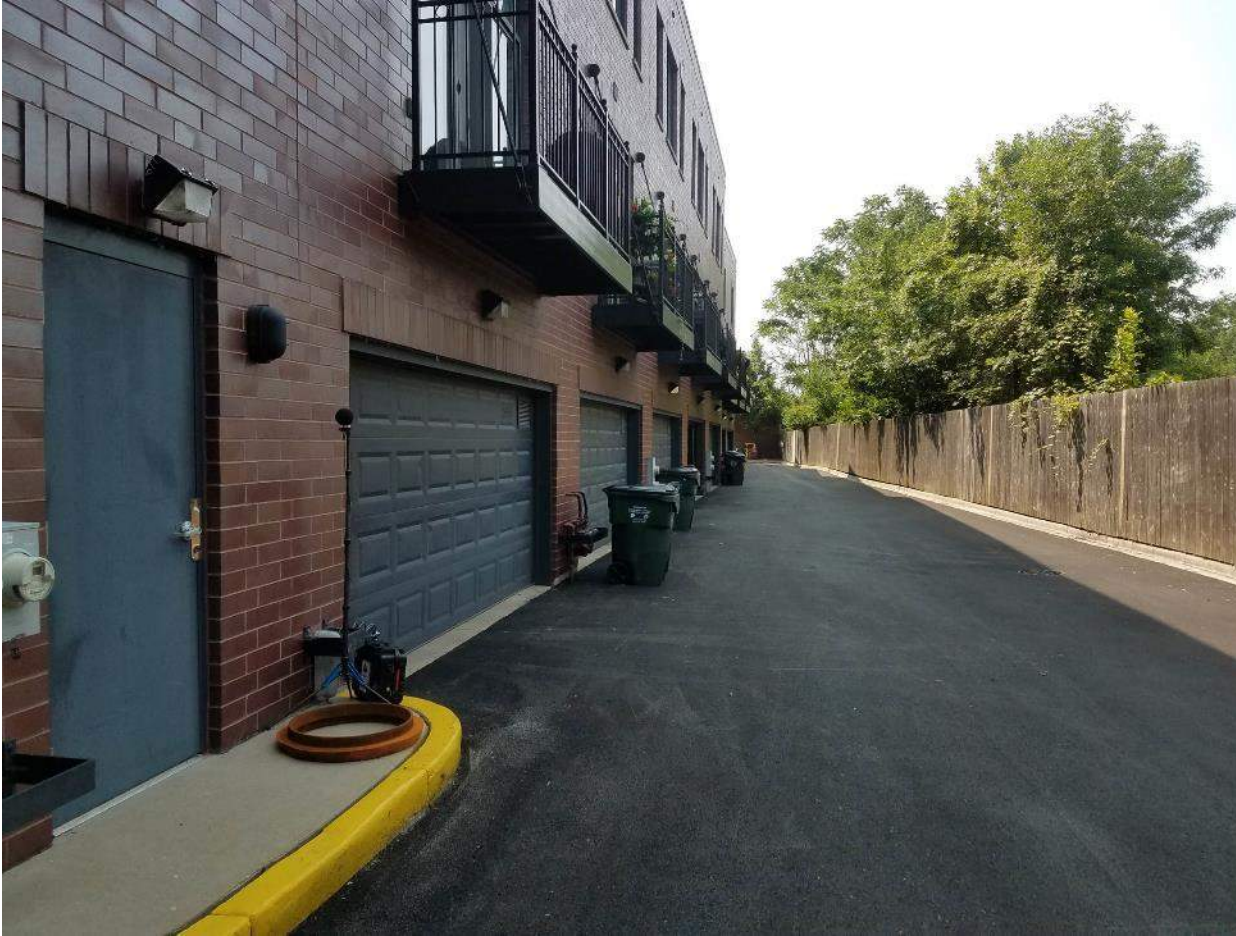
Figure A-9: Site LTN-9, 2654 N. Hartland Court, located on west side of residences, looking south toward Metra tracks
