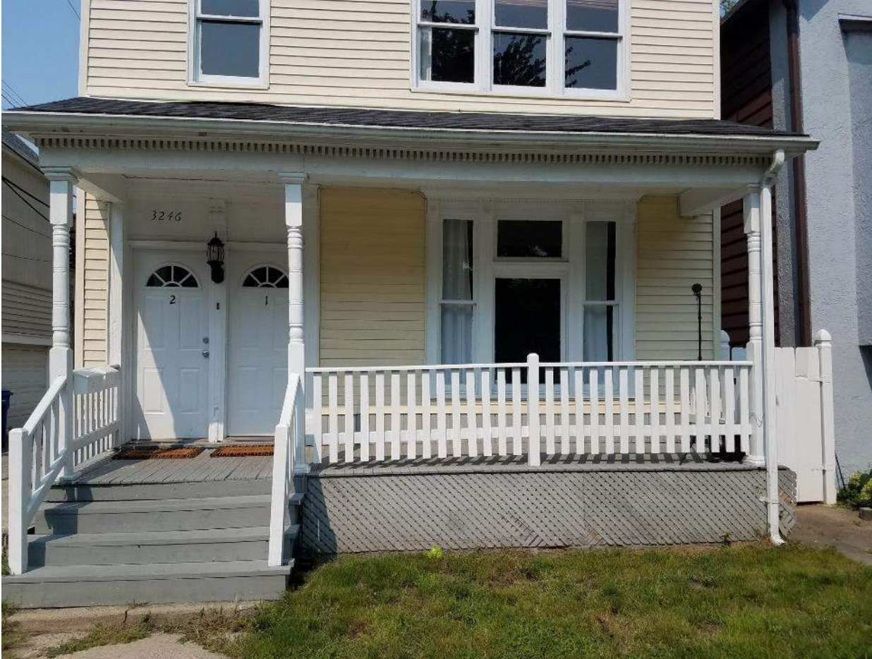
Figure A-4: Site LTN-4, 3246 N. Ravenswood Avenue, looking north toward residence, located west of Metra tracks
