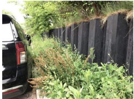
Metal Sheeting Photo by J. Mengler
