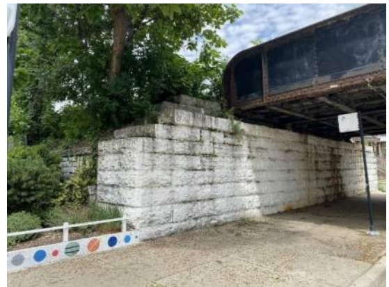
Masonry Abutment Photo by E. Stoner
