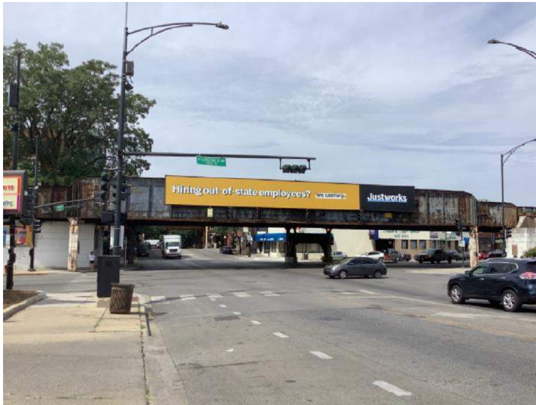
Figure 3-7: Lincoln Avenue/Addison Street Bridge
