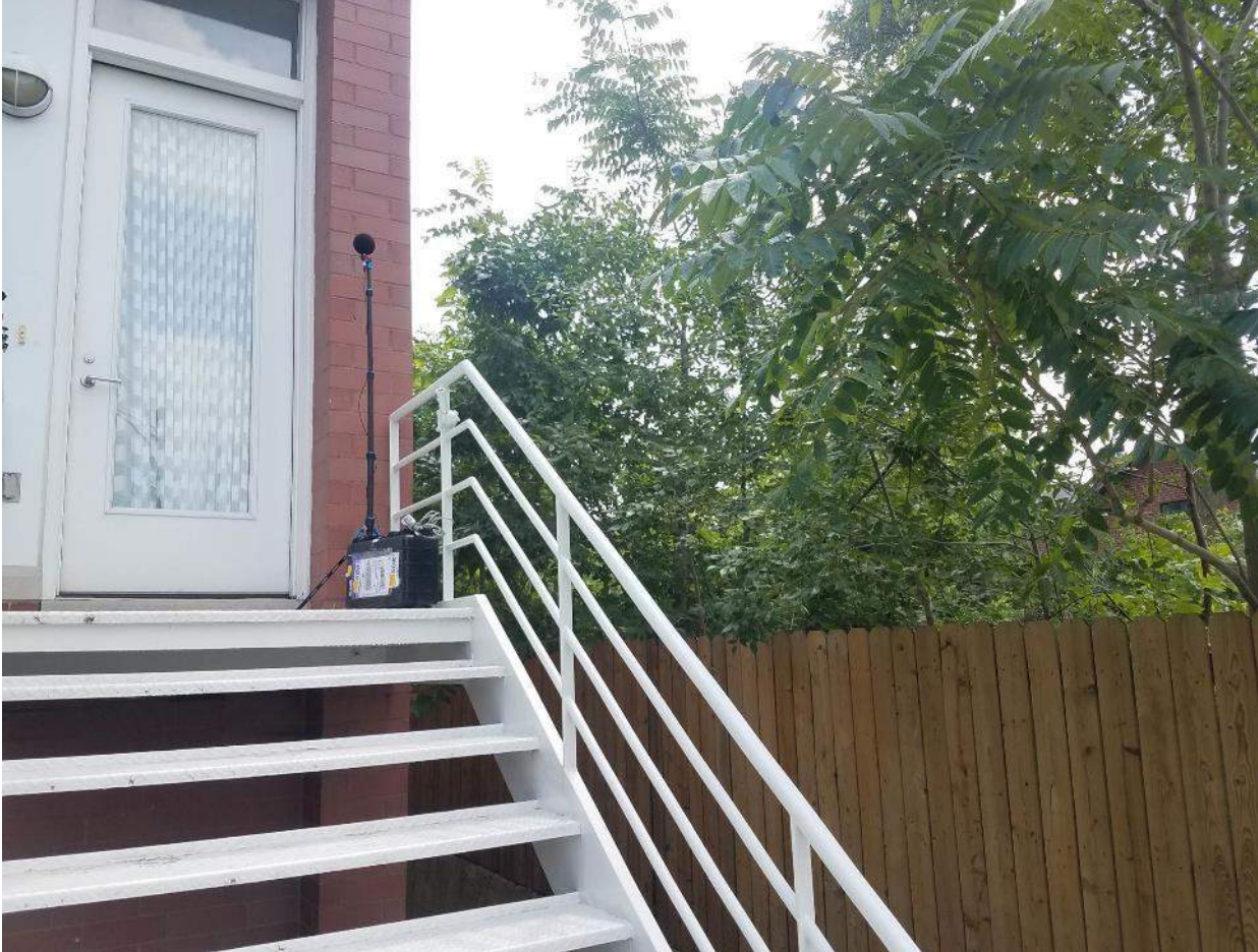
Figure A-7: Site LTN-7, 1763 W. Wellington Avenue, looking west toward Metra tracks
