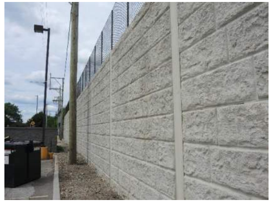
Concrete Retaining Wall Photo by S. Hands
