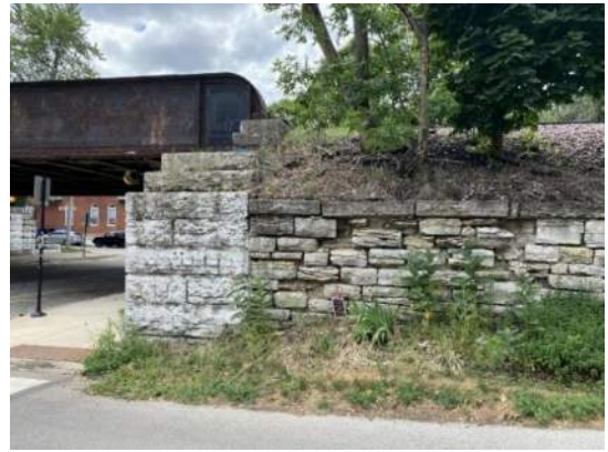
Stone Retaining Wall Photo by E. Stoner
