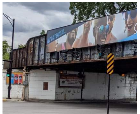
Concrete Abutment Supporting Addison/Lincoln Street Bridge Photo by S. Hands
