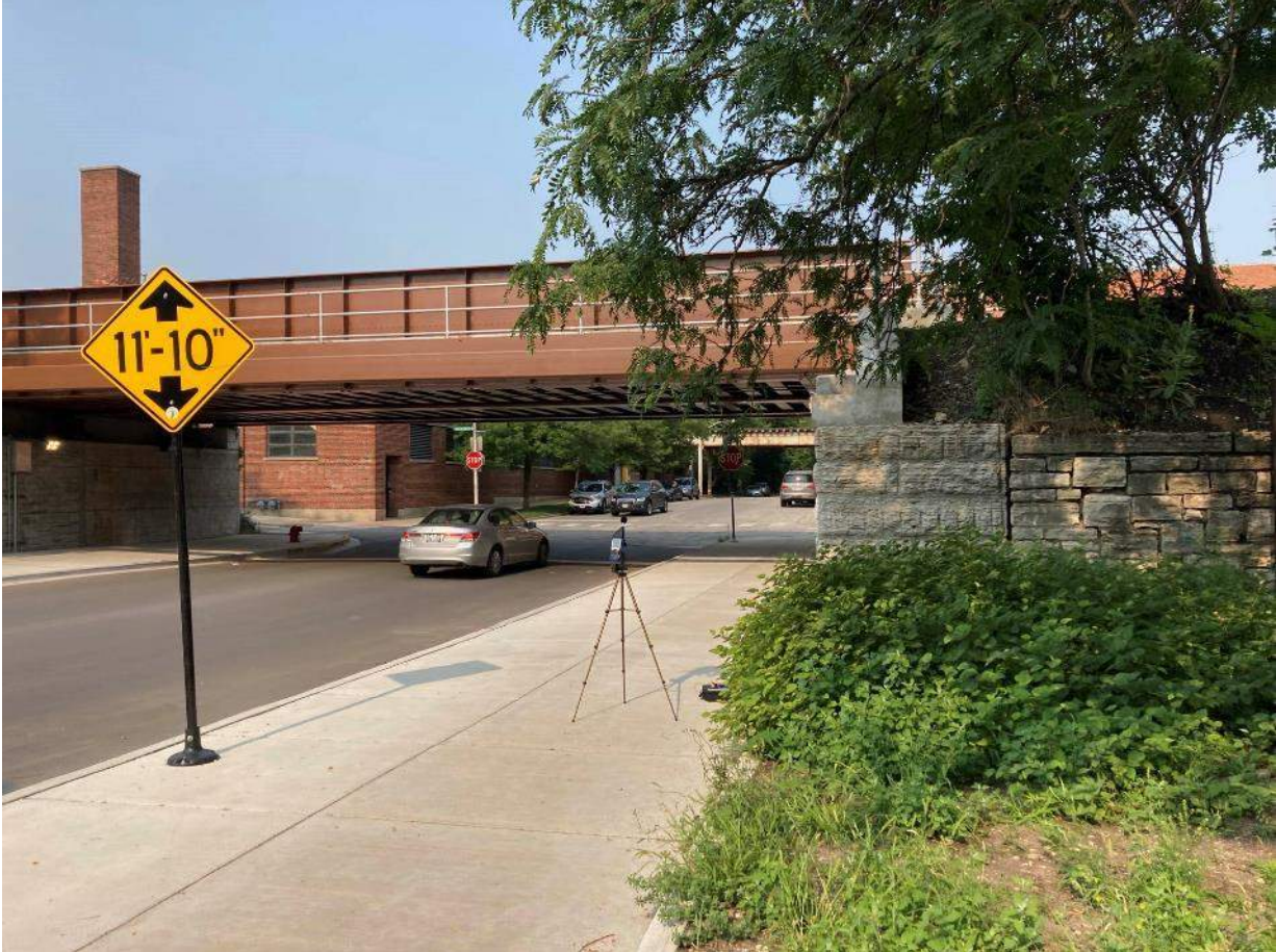
Figure A-12: Site STN-1, W. Berteau Ave. Metra Bridge, looking west toward Metra and CTA tracks
