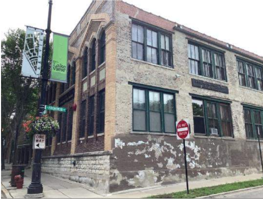
Figure 3-12: 1751-1757 W. Belmont Avenue, Secondary Elevation
