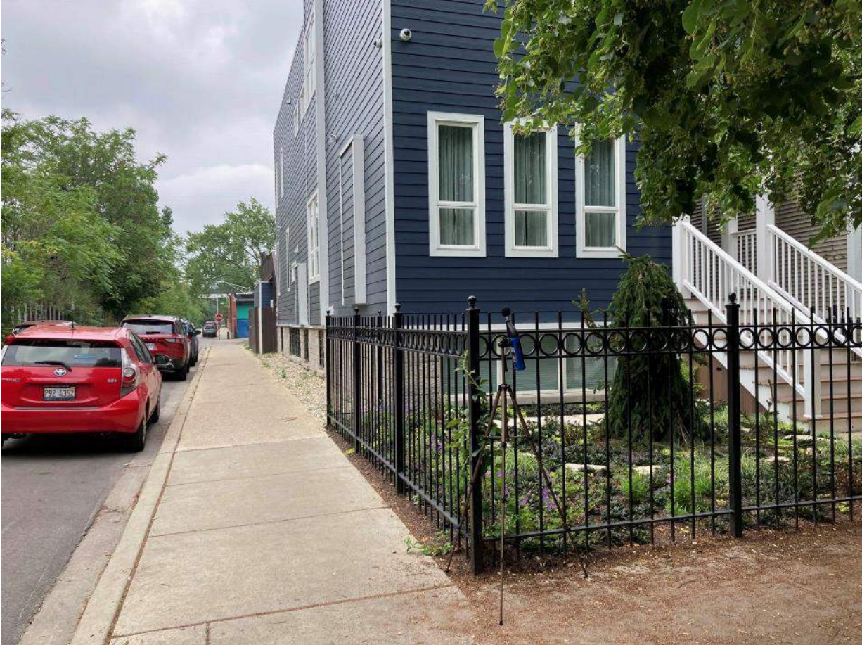
Figure A-18: Site STN-7, 1801 W. Eddy Street, looking north from W. Eddy Street.
