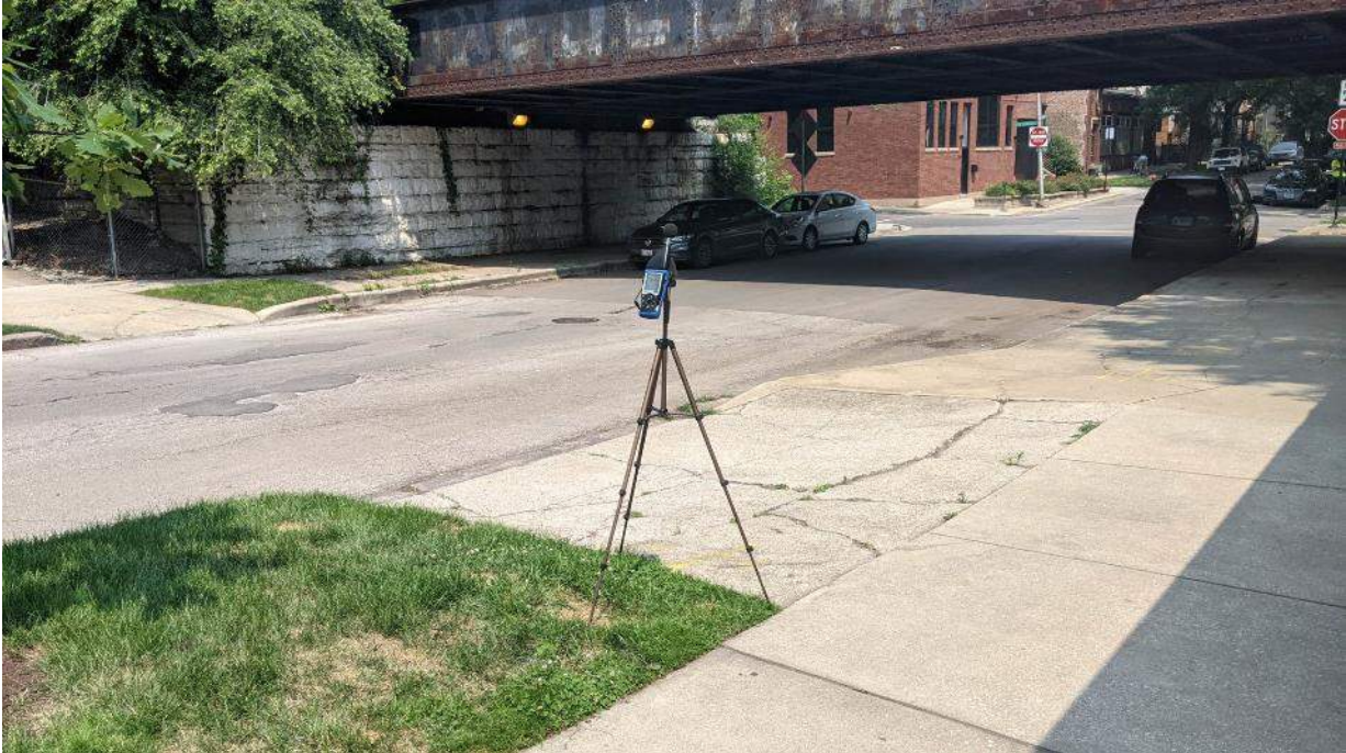
Figure A-15: Site STN-4, W. W. Barry Ave. Metra Bridge, looking east toward Metra tracks
