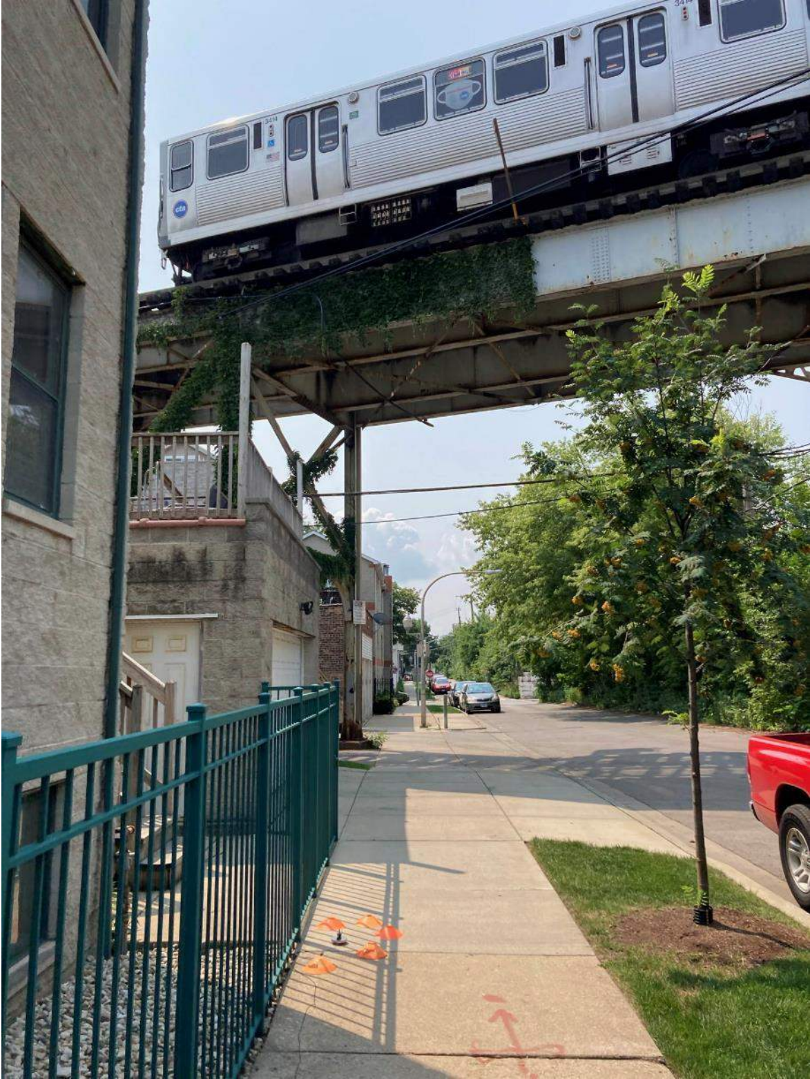
Figure A-23: Site STV-2, 1757 W. Newport Avenue, looking south toward CTA elevated structure
