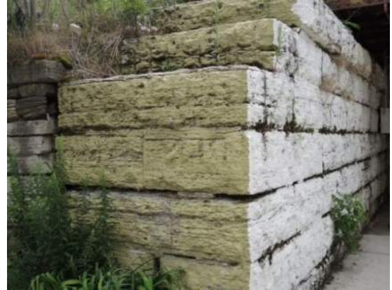
Masonry Abutment Photo by S. Hands
