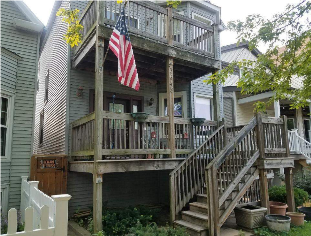
Figure A-1: Site LTN-1, 3645 N. Ravenswood Avenue, looking southwest from Metra alignment
