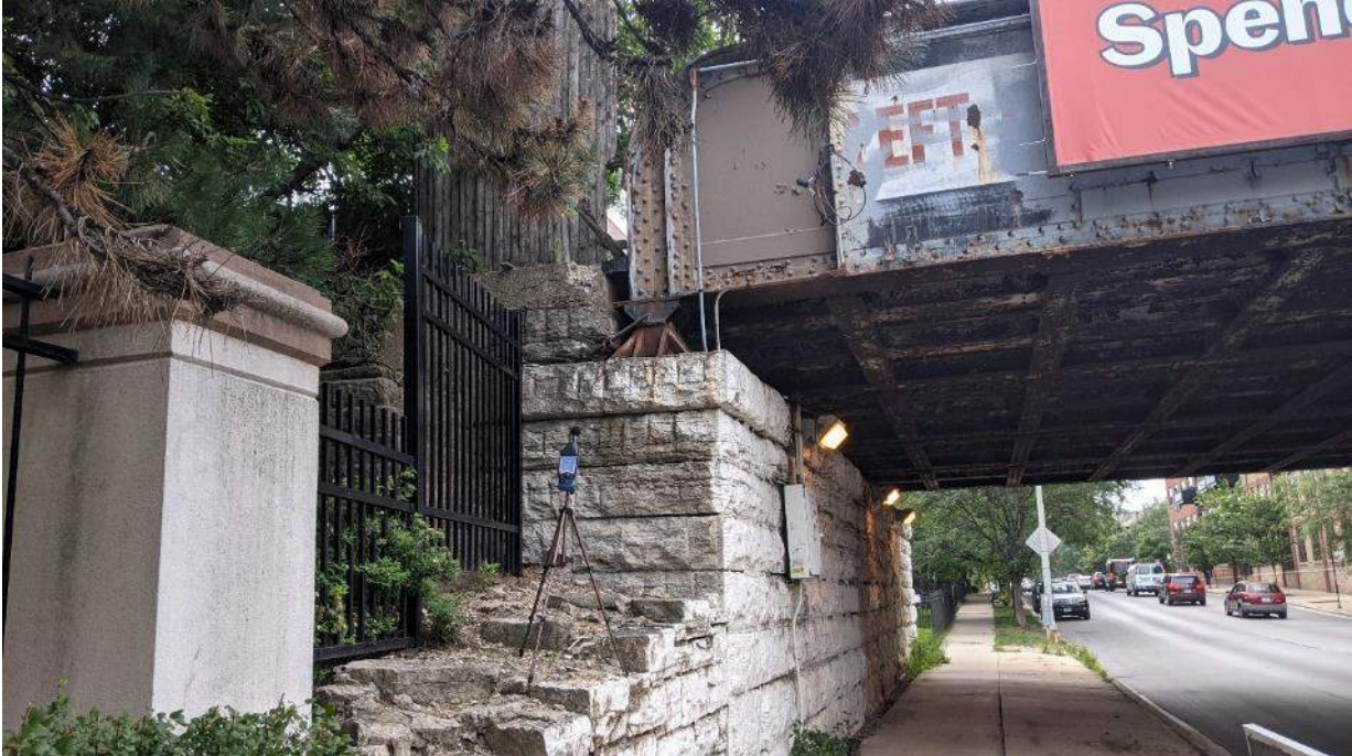
Figure A-21: Site STN-10, W. Diversey Pkwy. Metra Bridge
