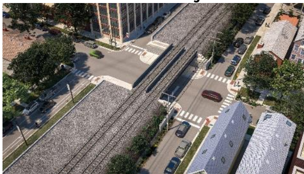
Unused Track #0 and bridge removal and west retaining wall installation.
