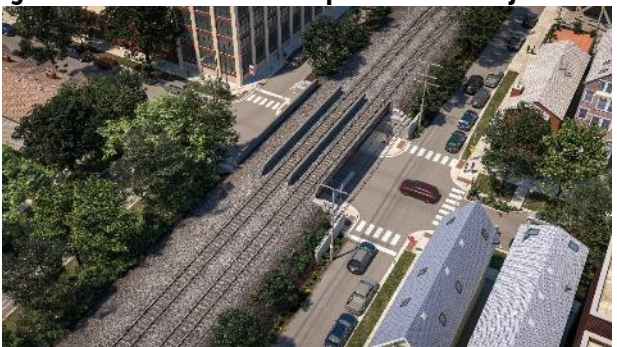
Existing track alignment along corridor.
