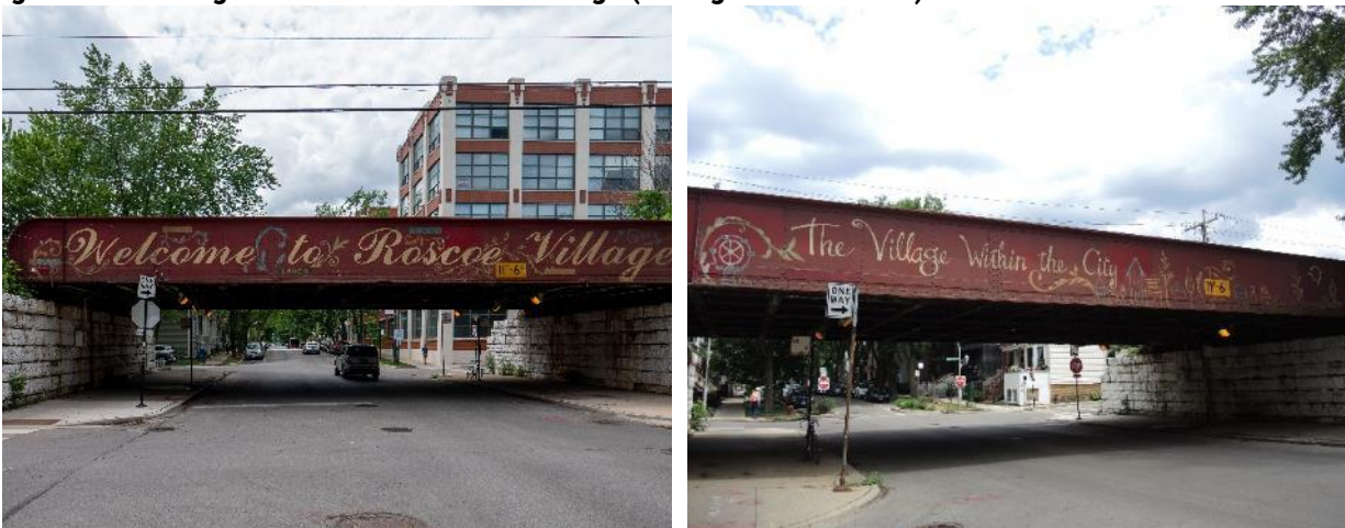
(Left) Roscoe Street bridge mural facing east; (Right) Roscoe Street bridge mural facing west
