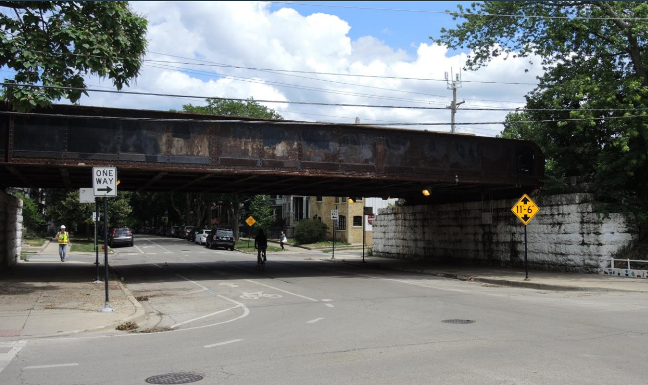
Existing Bridge at School Street
